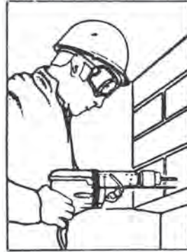
2. Digging holes in walls and ceilings
