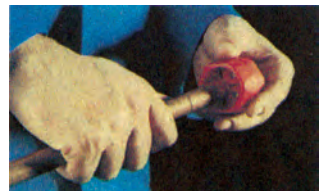
Removing the burrs with a reamer
