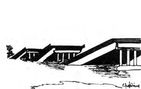
A bridge damaged by an earthquake
