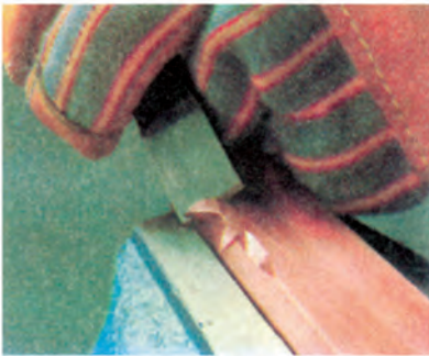
21 Scraping metal surfaces
